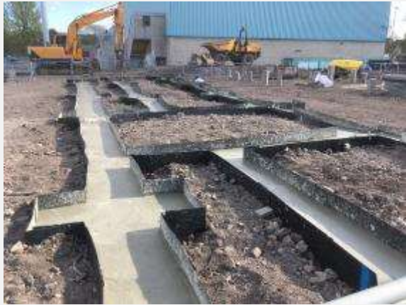
Foundations in Progress
