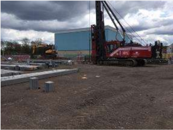
Piling Rig in Progress
