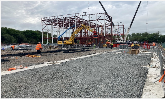
Foundations & steel frame in progress
